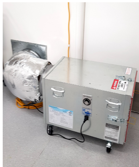
Image 1: The mini Condor© is installed in an operating theatre. It is capable of converting the normal positive room to negative pressure within seconds, when the unit is switched on.
